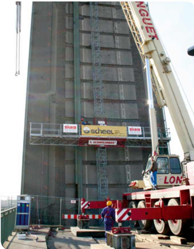
SC4000 lying with 7° slope used as single mast transport platform
